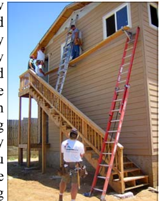
The siding is almost finished.
