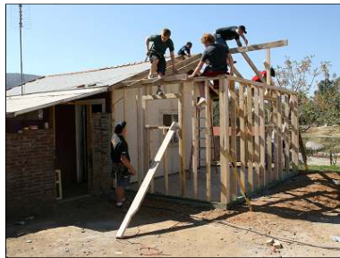
An addition gets framed.
