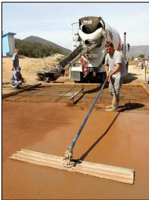
Ron Hager hard at work on the new driveway.
